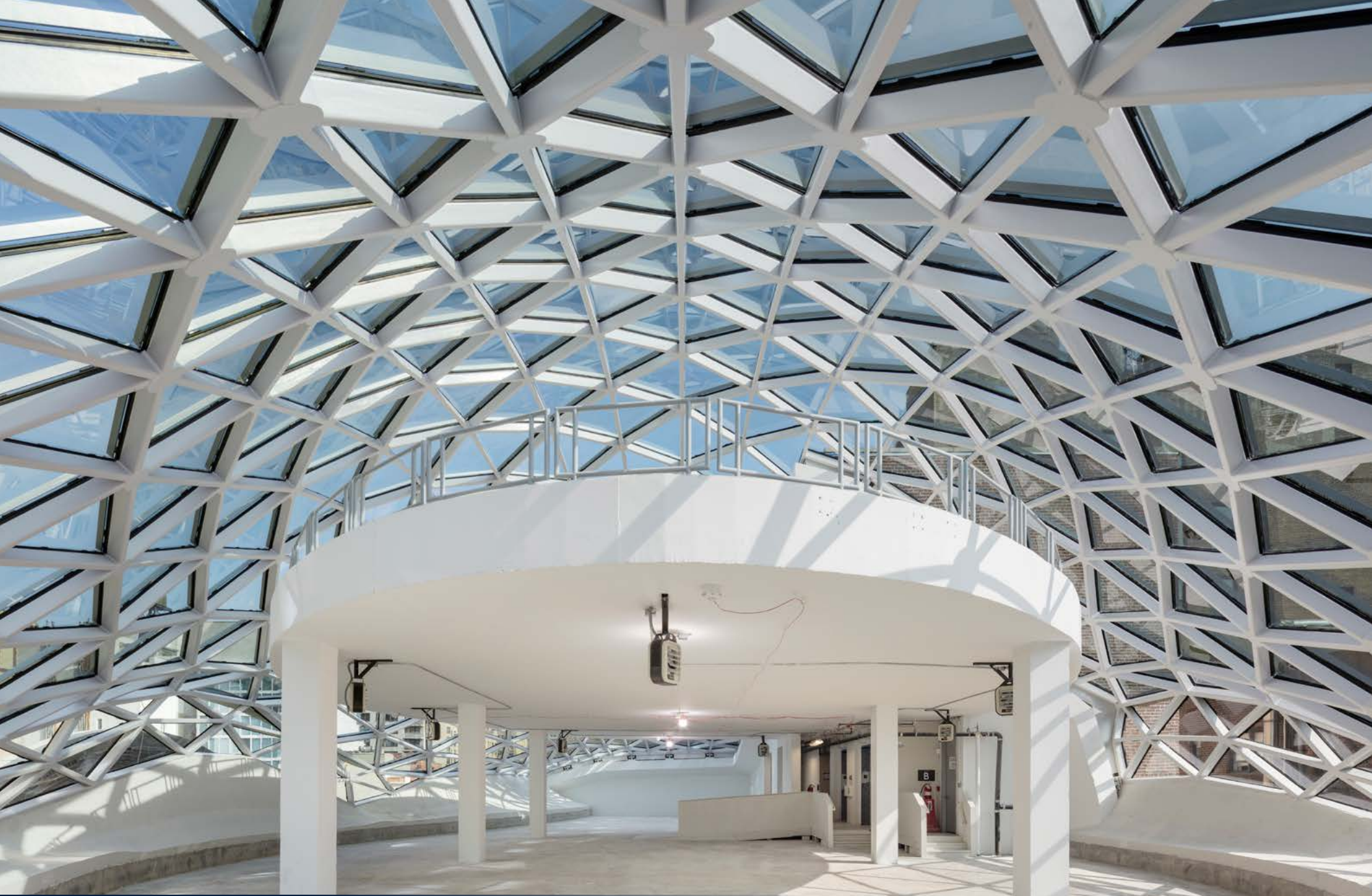
FIFTH FLOOR VIEW
